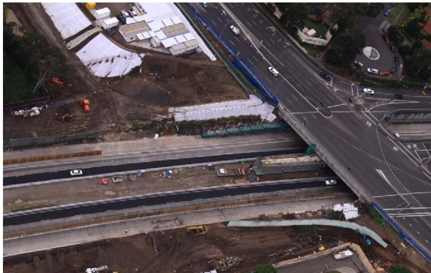
Windsor Road Bridge, Baulkham Hills 2 May 2011
