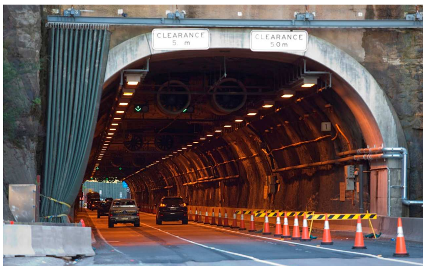
A noise curtain that has been installed on the western end of the eastbound Norfolk Tunnel
