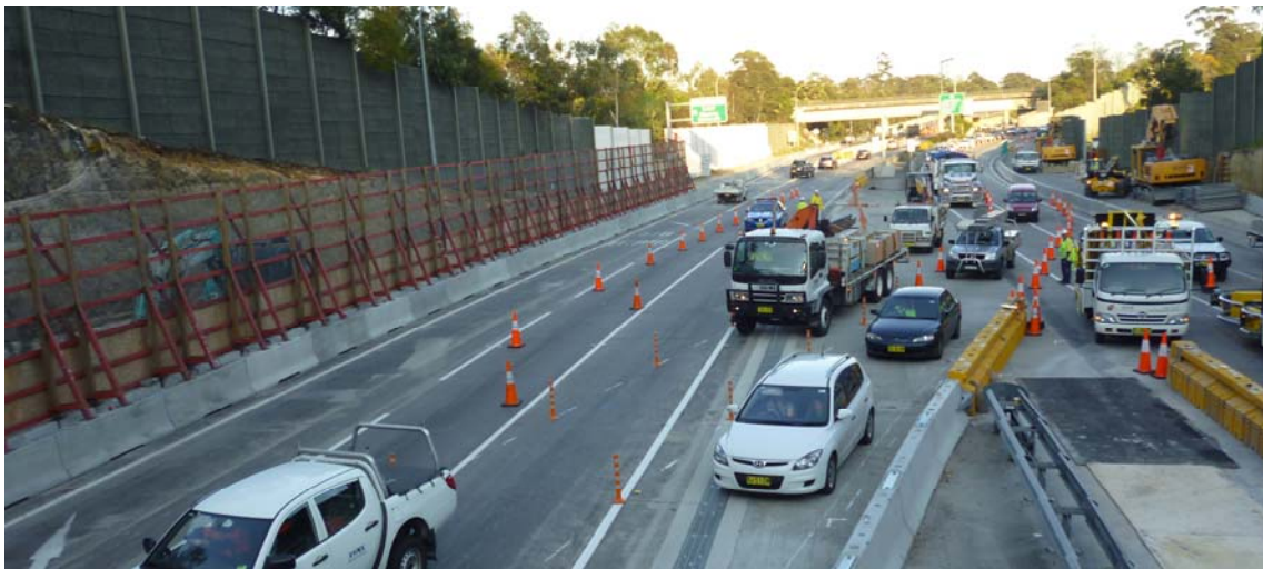
Contra flow in place west of the tunnel
