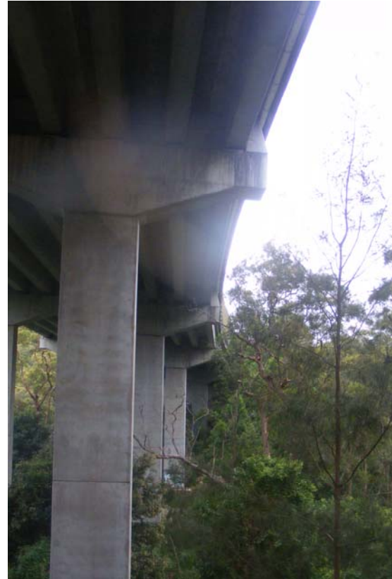
View from under Terrys Creek Bridge
