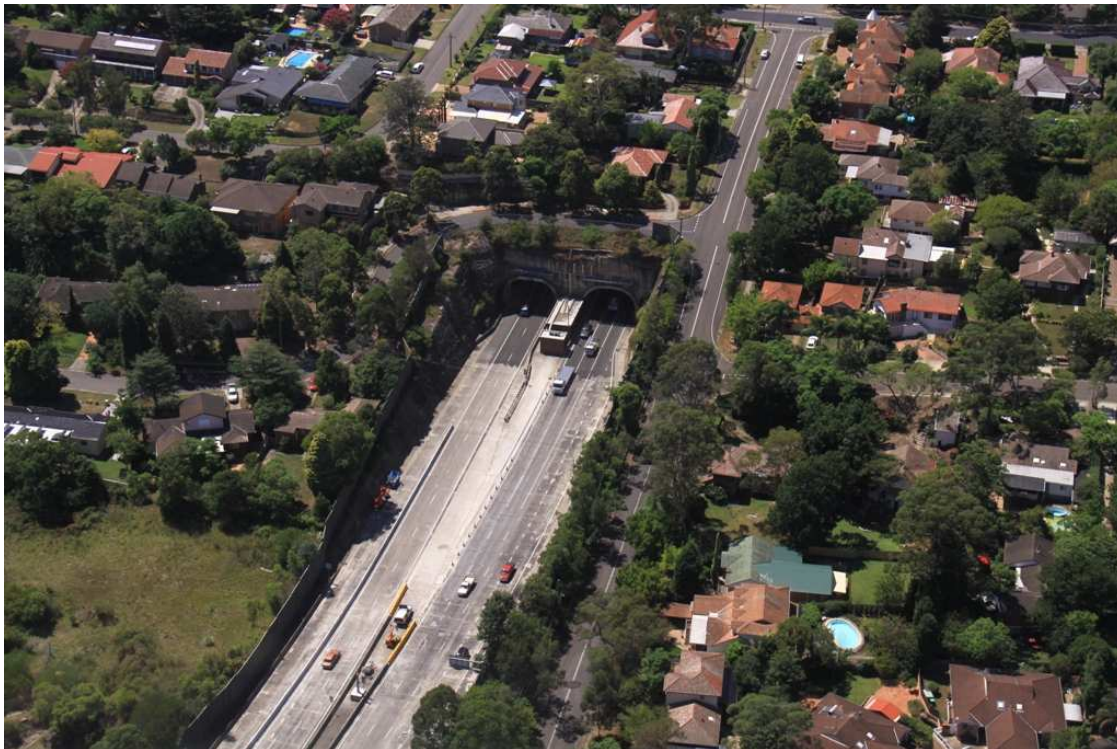
An aerial photograph of the Norfolk Tunnel western portal
