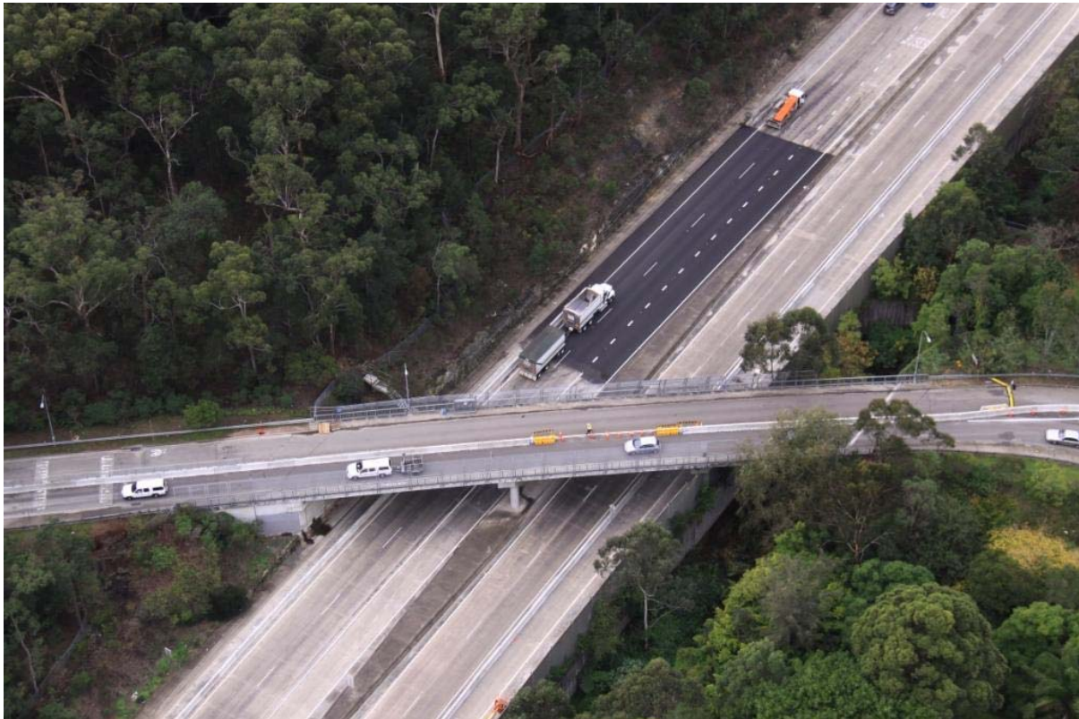
Murray Farm Road Bridge, May 2011
