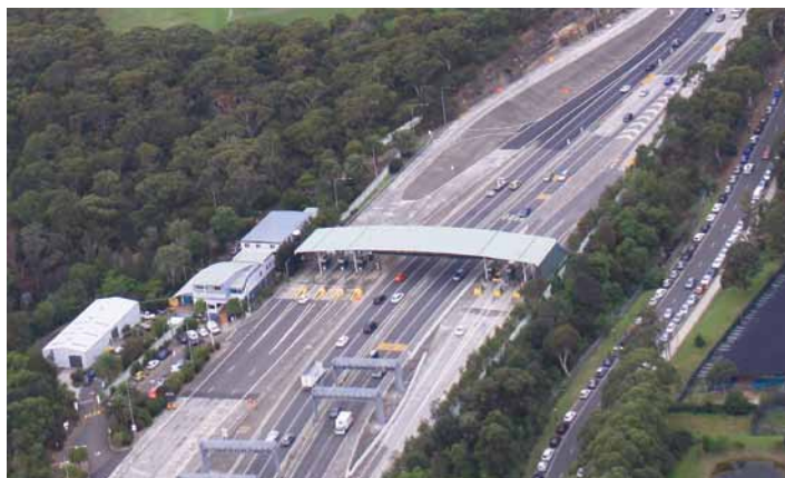
Toll plaza canopy at Macquarie Park, February 2011
