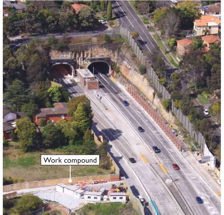
West of the Norfolk Tunnel
