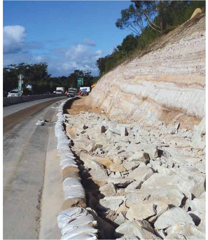
Erosion controls westbound, west of Murray Farm Road Bridge, Beecroft
