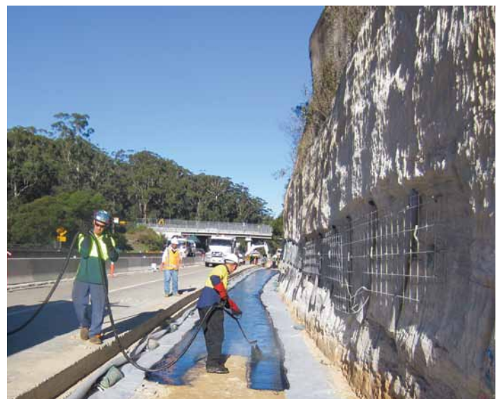
Spray sealing west of Murray Farm Road Bridge
