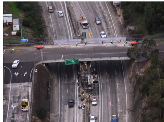
Christie Road Bridge over the M2
