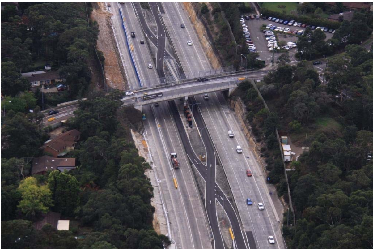
An aerial photograph of the M2 Motorway and the Barclay Road Bridge
